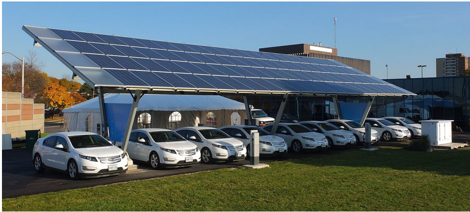
Fig. 1: Environmentally clean yet slow way of EV charging - direct usage of photovoltaic system[5]
